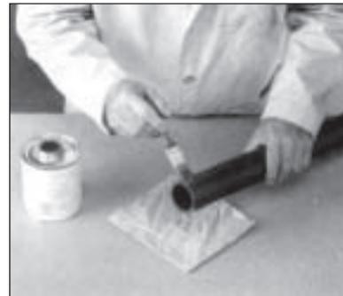
Apply a medium layer of cement to the fitting socket. Do not let the cement puddle. Also, when joining belled-end pipe, do not coat beyond the bell depth or allow the cement to run down the inside of the pipe.
