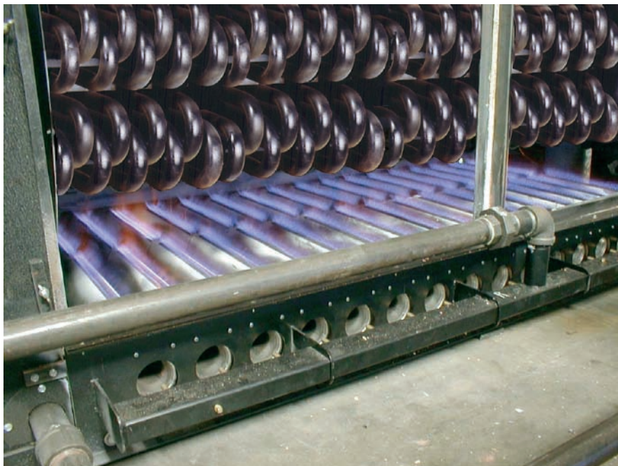
Parker Atmospheric Low NO x Burners Firing in a Parker 50LA Steam Boiler
