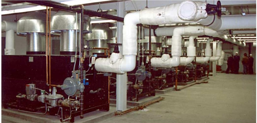
*The Parker bent steel tube, all welded construction is the ideal boiler for high temperature applications. Pictured is the Boiler Room at HMT Technology Corp. in Eugene, Oregon. Here, four T-4600's provide the heat source for a metal plating line (350°F), and three T-6800's serve the building heating needs of the facility.*
